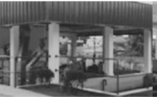
Carmona WATER DISTRICT 20 m 3 /day
